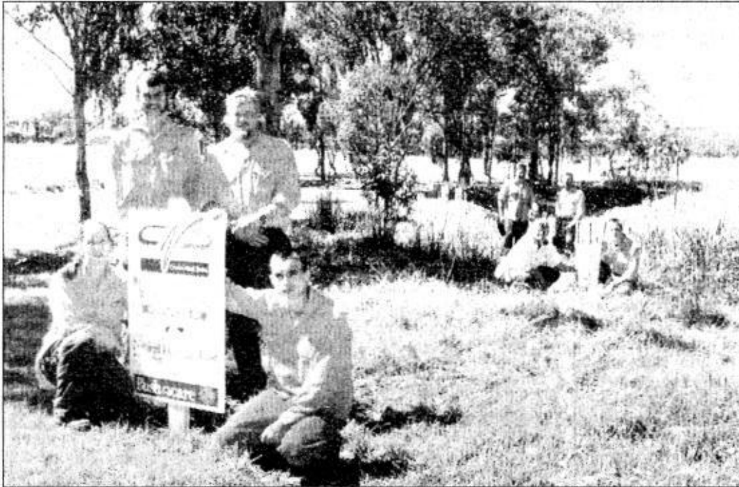
WATERCOURSE WORK: Crows Nest Shire Council Natural Resource Management field supervisor Steven Plant (front right) supervises seven trainees on the job at the Charles Street Water Course as they work to stabilise the creek bank to prevent it washing away in the event of heavy flooding. With Mr Plant are (standing left) Doug Ashford, (kneeling) Maleena Sutton and Matthew Gower, (right back) Matthew Rebb and John Morrison, (right front) Steven Carter and Alistair Crawford.
